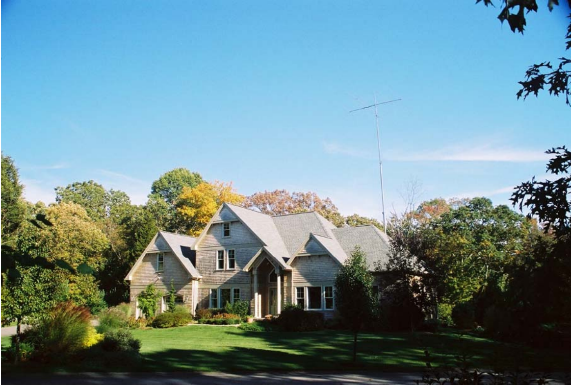
Home of K6JRY, antenna up. Photo shows a US Tower, Model MA-770MDP (the motor drive version), which nests to ~23'. Fully extended, it can reach (without additional mast) 71'. The foundation is 5' x 5' x 5' of reinforced concrete.
