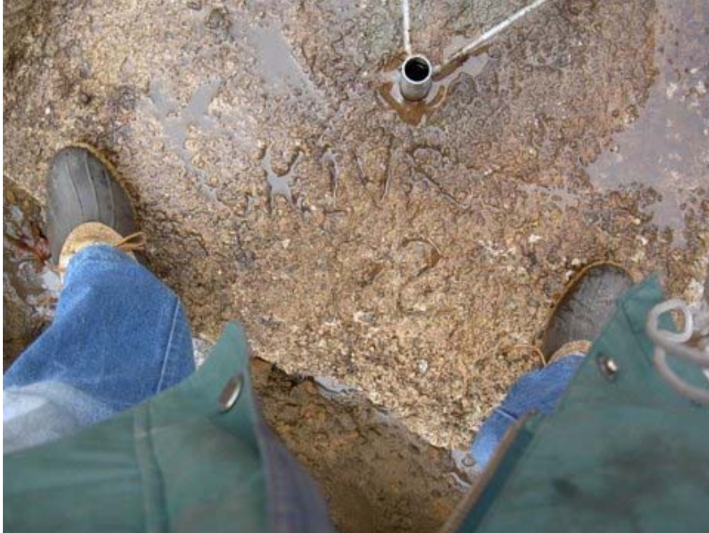
Figure _____. Written with a stick, the inscription in this base reads: “K1VR 82”. But does it really prove that the concrete was poured in 1982?
